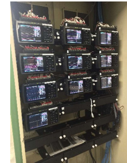
GL840 Embedded on cabinet
